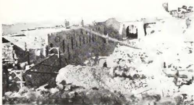
Fig. 3. Fort Daspoortrand under construction (T.E. Andrews Collection).
